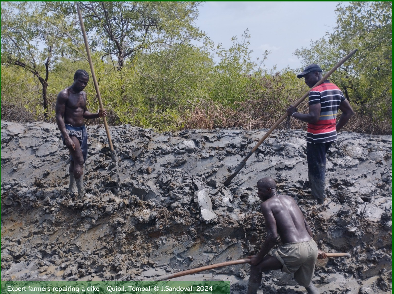
Expert farmers repairing a dike – Elalab, Cacheu © J.Sandoval, 2024
