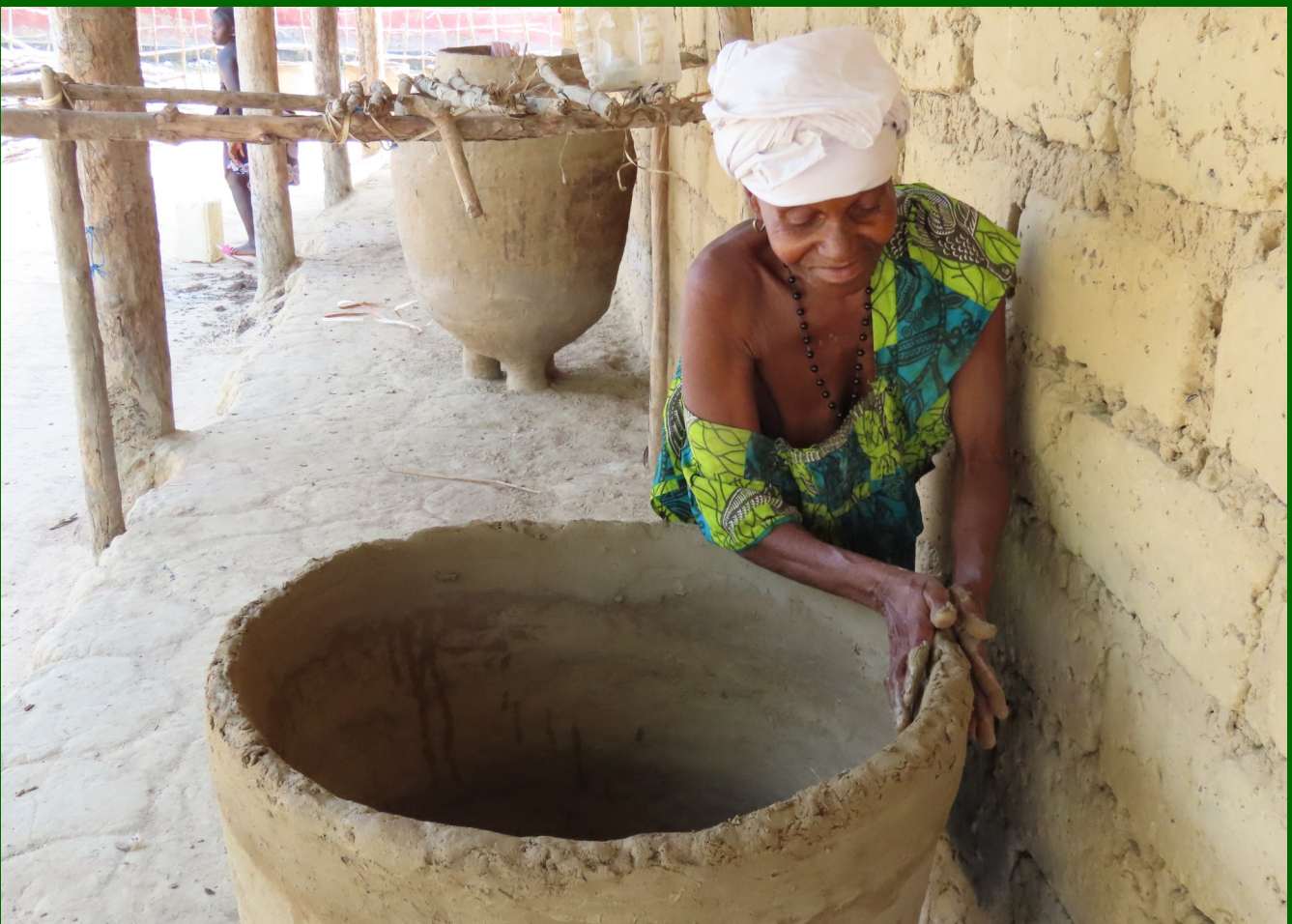
Old woman building a bowl-silo ( fuúle/vuúle ), layer by layer as it dries – Cafine, Tombali © S.Conde, 2022
